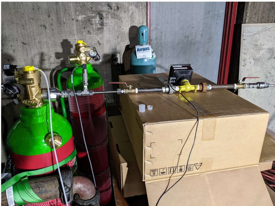
Figure B6 –NOVEC cylinder with Connected pressure transducer and flow meter– only one cylinder was used and the other cylinder near the wall was a spare cylinder.
